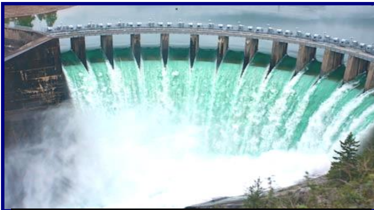
Kerr Dam in the spring and fall
