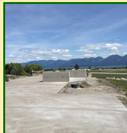
Construction at Site #176
